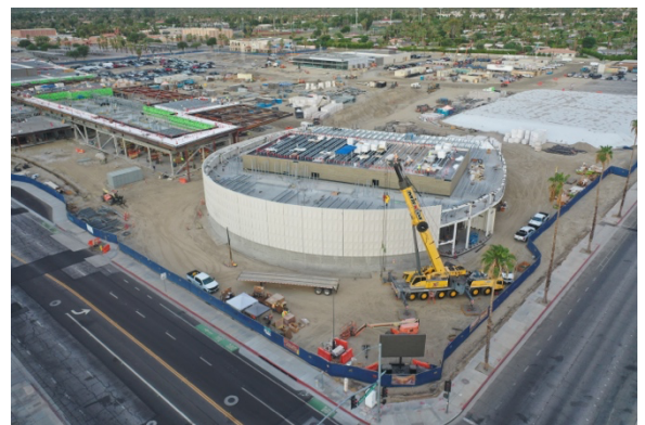
Photo: New three-dimensional architectural cladding wraps the Event Center at College of the Desert's Palm Springs Campus, creating a distinctive pattern of desert light and shadow at Tahquitz Canyon Way and Farrell Drive.
